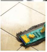
"Post-installation" cleaning helps remove residues of joint grouts, cement and lime. This operation is mandatory after installation both for glazed and unglazed tiles. Never clean tiles that are too hot (e.g. exposed to sunlight during hot summer months) since the reaction of aggressive chemicals may become harsher. In the summer, proceed with the operation during the coolest period of the day.
